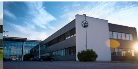
EV R&D Center, Kottlingbrunn, Austria E-drive systems and transmission development
